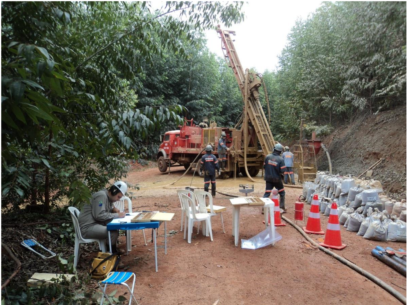
Figure 9 – Geosedna RC Rig drilling at Jambreiro Project
