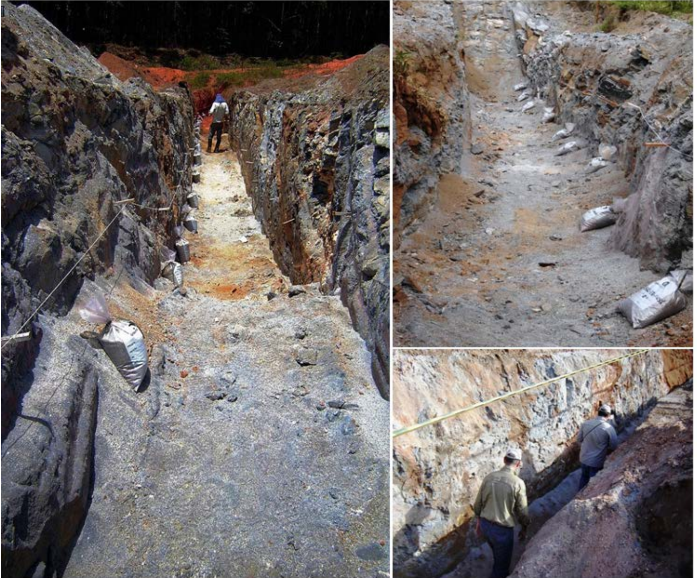
Figure 3 – Photos Showing Trenching across the Ore Zone at Tigre Prospect, Jambreiro
